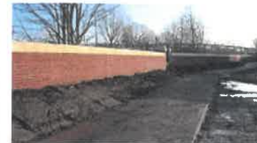
Example sheet pile wall with timber coping
